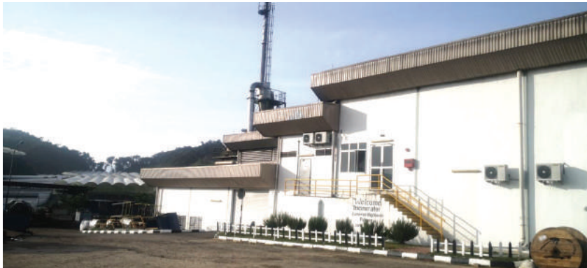
Cameron Highland 40 Ton/Day Incinerator.
