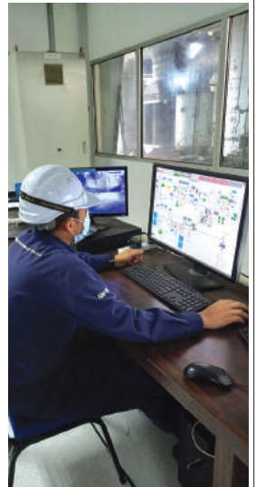
View from Control Room.
