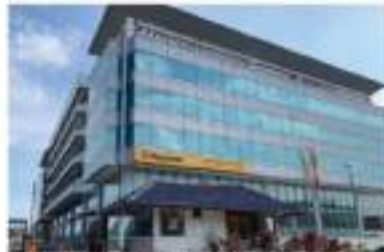
Maybank Group Customer Care (MGCC), Bukit Jalil, Shah Alam
